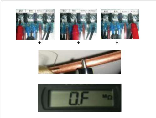
CH 05/53 (Indoor/Outdoor Device Communication Error) → Detection by indoor devices
