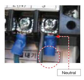
(4) Communication noise by oxidized wire arrangement: Soldering is required.
