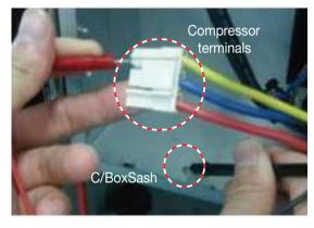
Measure the resistance between a compressor terminal and panel.
